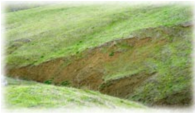
Above: Unstable hill slope in spring 2002.
